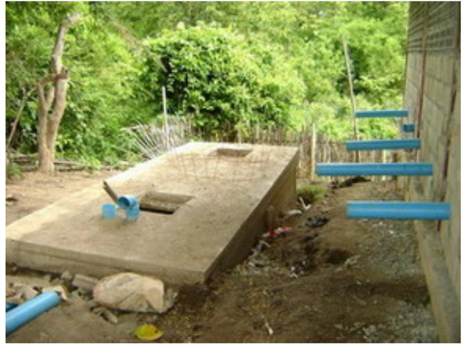
Backside with sewer pipes leading to two large septic tanks behind boys' toilet & shower area
