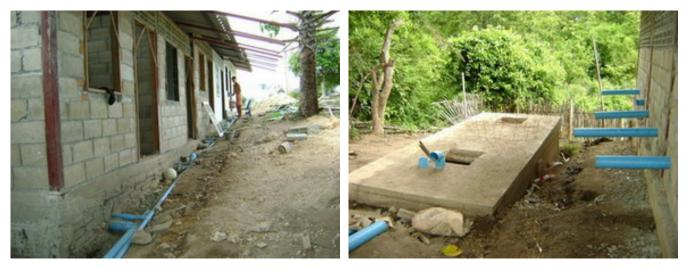
Backside with sewer pipes leading to two large septic tanks behind boys' toilet & shower area
